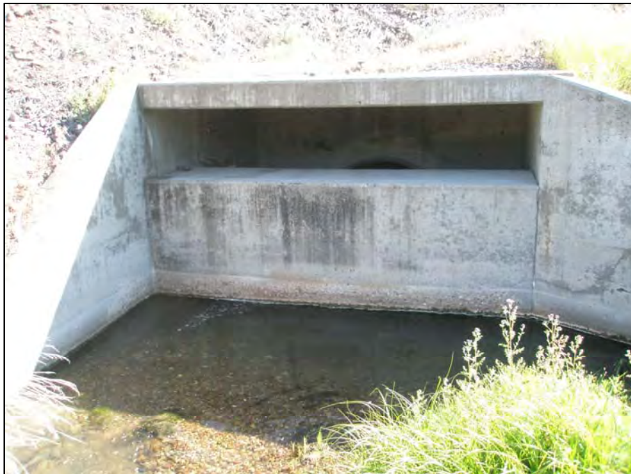
Photo C2 outlet of I-90 culvert looking at energy dissipater
