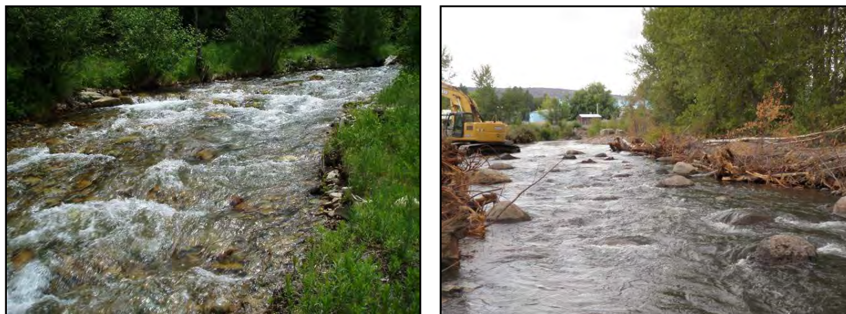
Figure 3-1. Example constructed channels incorporating graded alluvium and boulder placement for grade control and aquatic habitat diversity.
