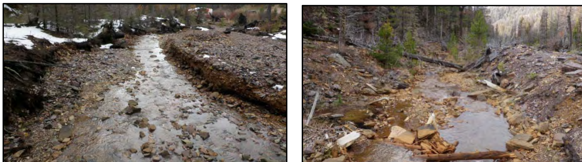
Figure 2-6. Existing valley and channel conditions in Reach 3, Lower Beartrap Creek. This reach is affected by large quantities of sediment transporting through the system, in addition to erosion from adjacent hillslopes.
