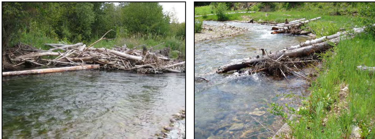
Figure 3-3. Photographs demonstrating the use of engineered log jams used in conjunction with streambank bioengineering structures and submerged wood to form a stable, vegetated land-water interface and create complex aquatic habitat along the channel margins.
