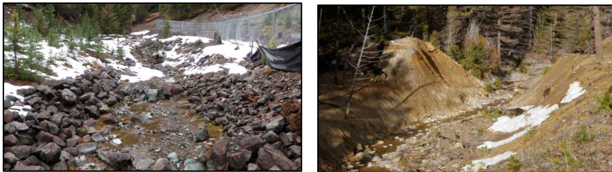
Figure 2-1. Existing valley and channel conditions in Reach 1 Mike Horse Creek. The upper reach (left photo) has been extensively armored and stabilized with rock. Downstream of Mike Horse Road, the channel is highly unstable and characterized by mass wasting features that contribute large volumes of sediment to the channel network (right photo).
