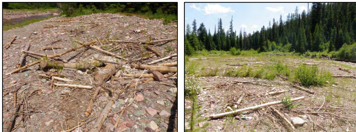
Figure 3-2. Floodplain woody debris and microtopography treatments are shown in the left photo. The right photo shows willows growing from buried cuttings combined with coir logs to sustain rooting zone moisture.
