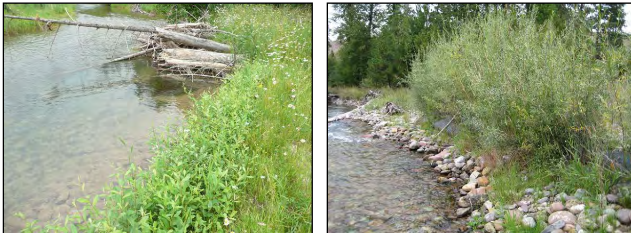
Figure 3-4. Vegetated soil lifts used in conjunction with engineered log jams (left) and as a stand-alone treatment (right).
