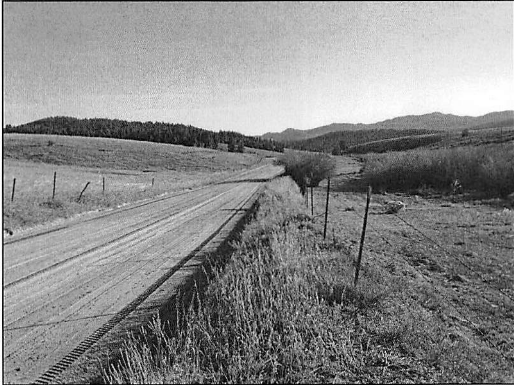
Site for New Basin Creek Water Treatment Plant
