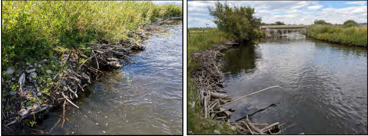
Figure 10. Left - Example of brush matrix providing overhanging cover and willows colonizing the face of the treatment (Phase 5). Right – Example of brush matrix with high woody cover behind bank and undercutting.
