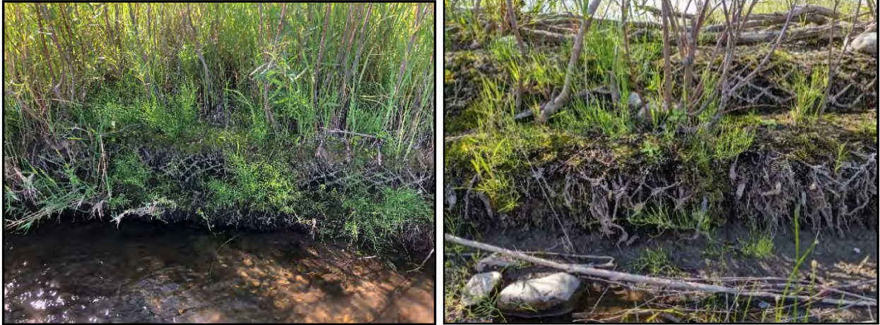
Figure 9. Left - Example of vegetated soil lift coir fabric and coir log being replaced with woody vegetation and colonized by herbaceous wetland vegetation.
