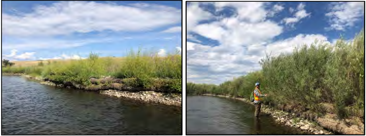
Figure 7. Soil lifts with cobble toe preventing undercut bank formation.
