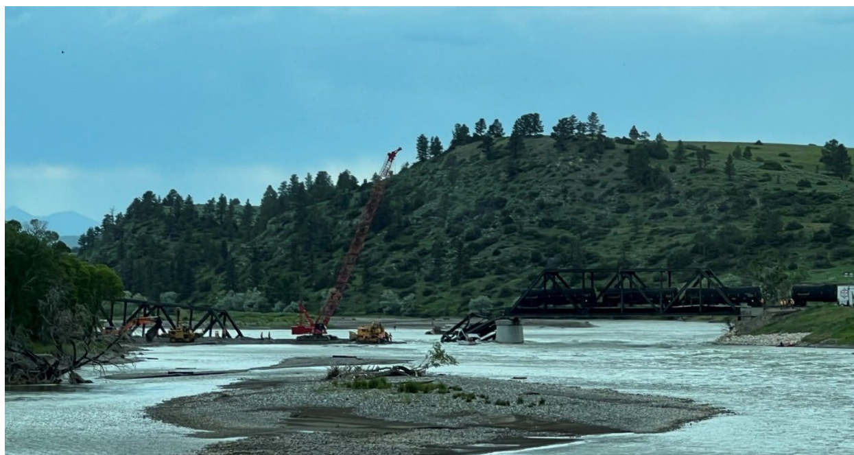
Exhibit 1-2. Side view of the Twin Bridges Road railroad bridge after the derailment.
