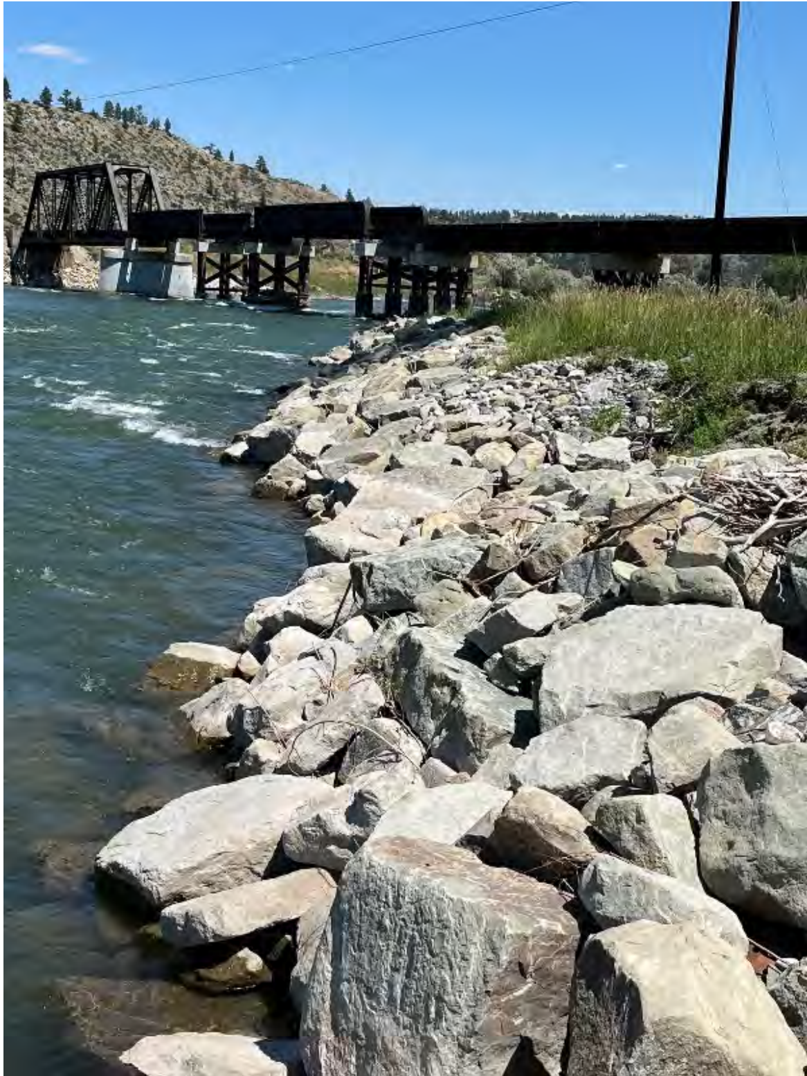
Bridge 51 riprap facing downstream (south-east) July 9, 2024.
