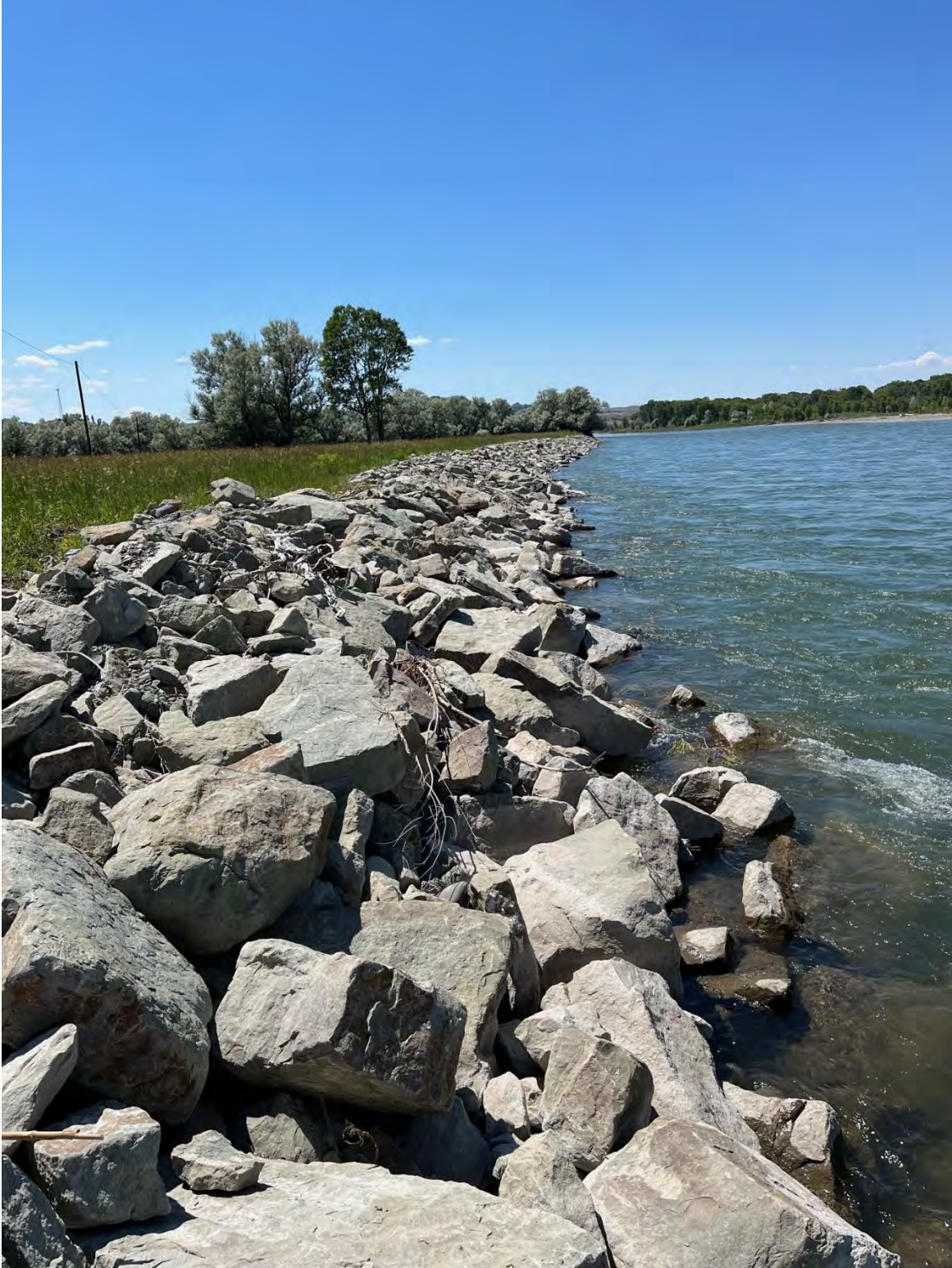
Bridge 51 riprap facing upstream (north-west) July 9, 2024.
