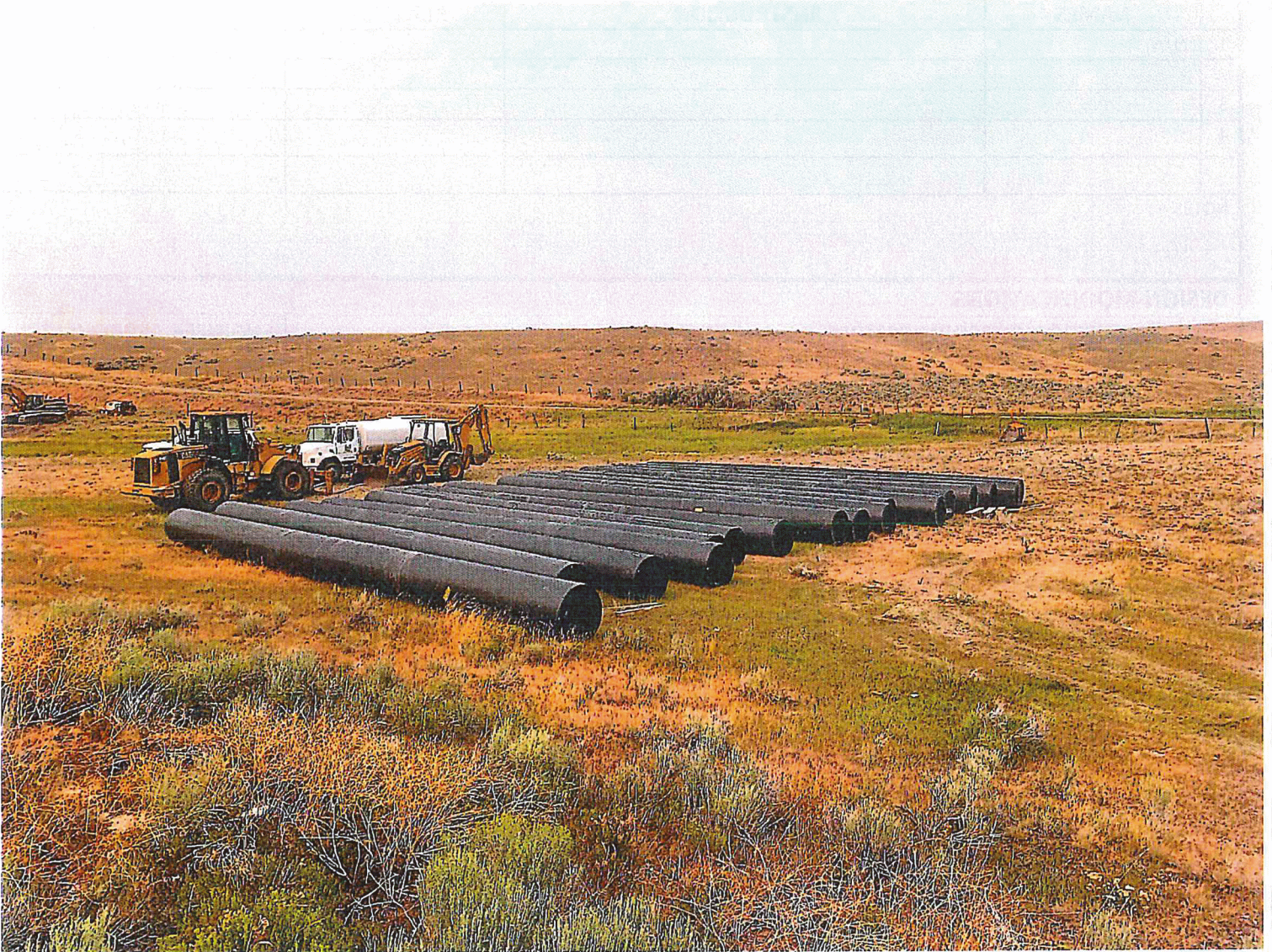
Stage 36" HDPE pipe at Frontage Road site
