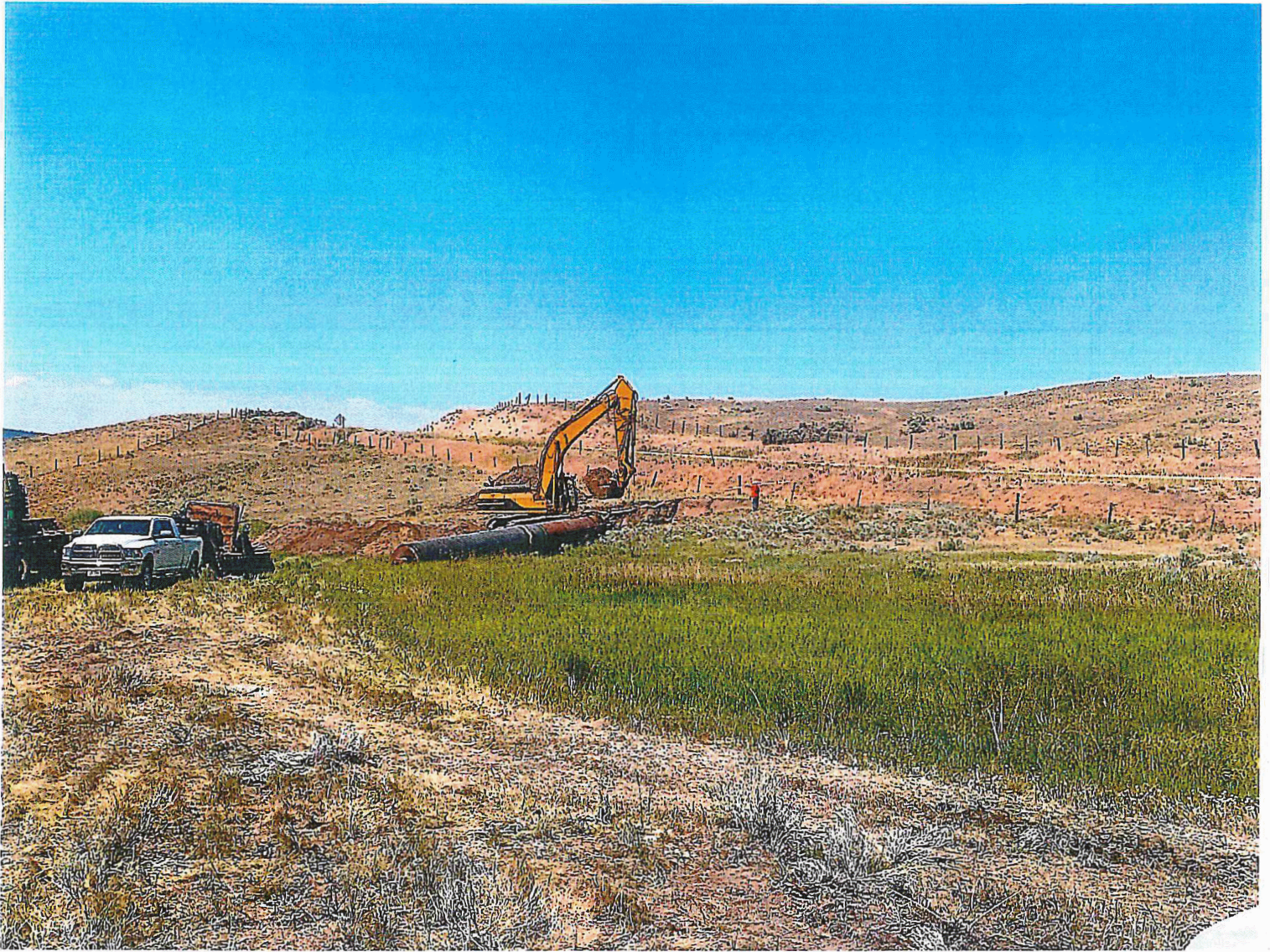
Coleman Construction beginning to construct Frontage Road bore entry pit near station 32+35
