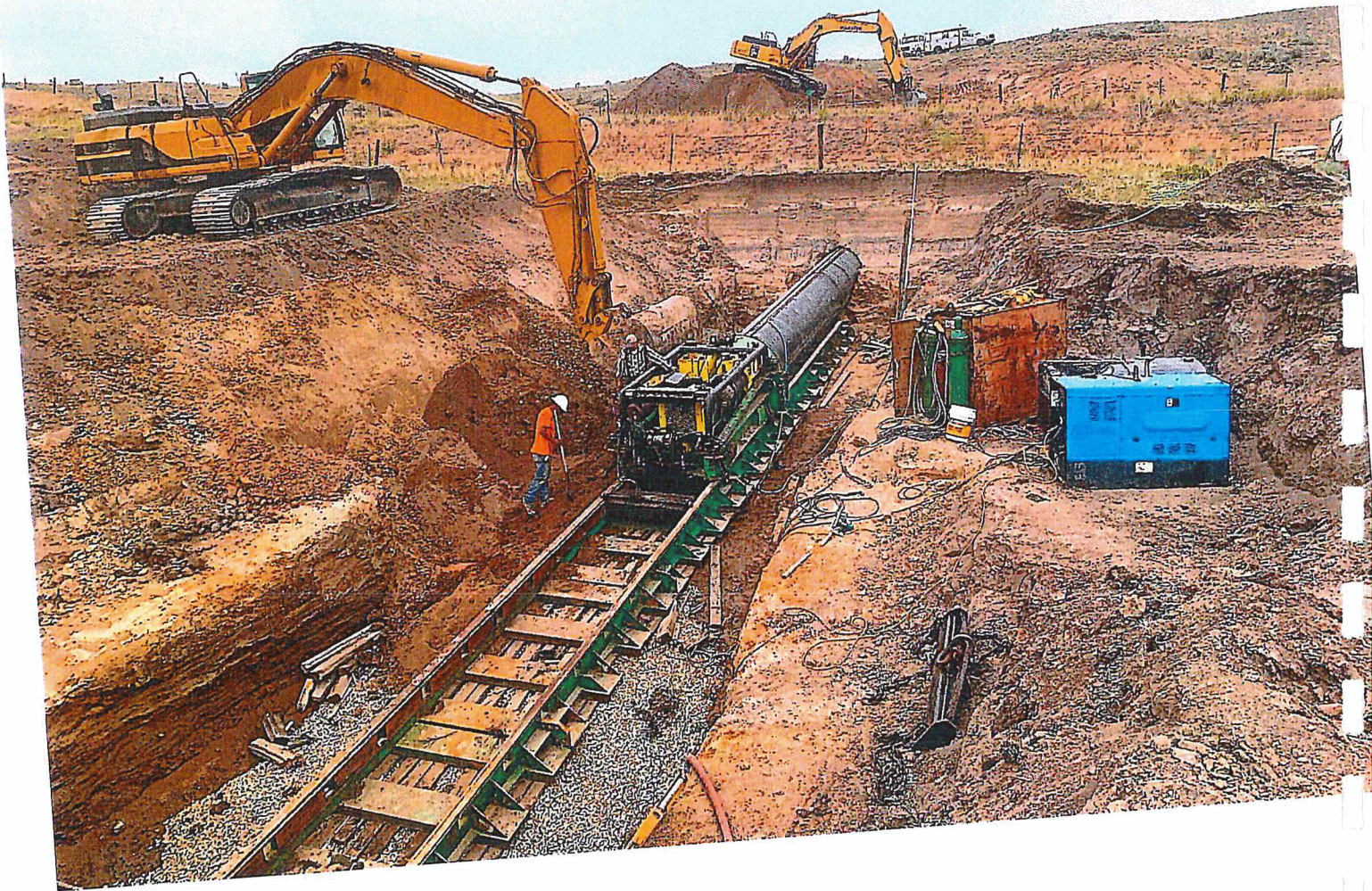
Installation of 48" steel casing at station 32+35
