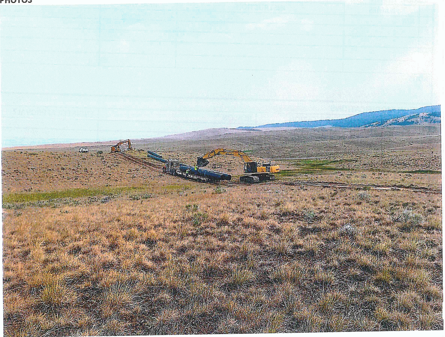
H&H contracting staging 36-inch HDPE pipe along alignment
