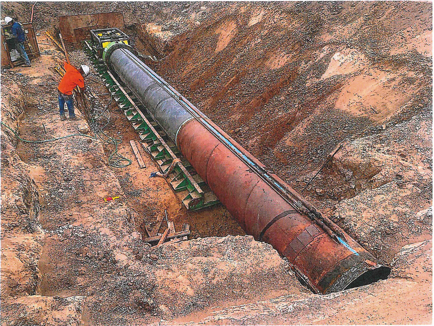
48" steel casing prepared for Jack and Bore installation at station 32+35
