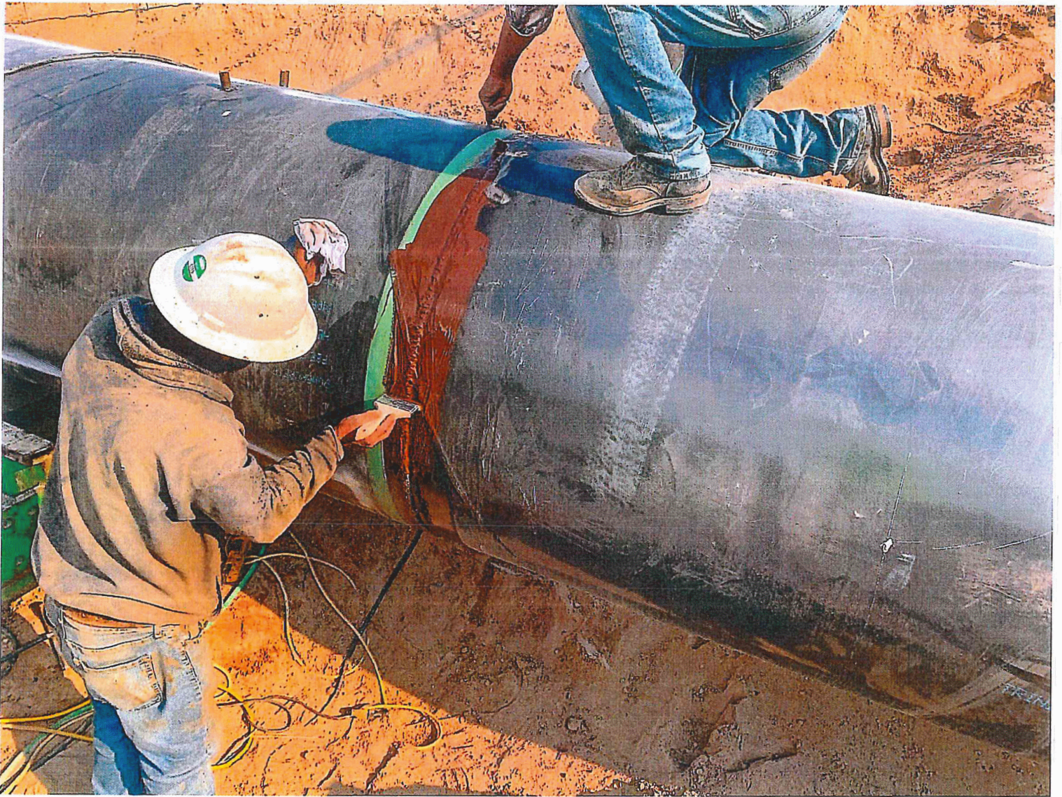
Coleman Construction applies Powercrete J to welded casing at station 28+63
