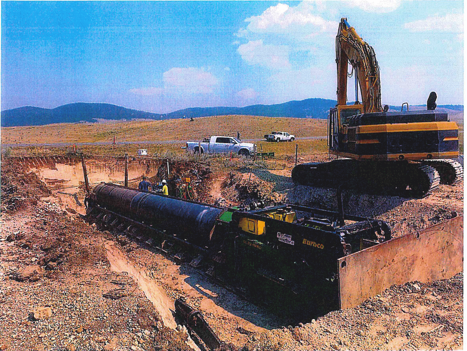
Coleman Construction excavates prepares for I-15 South Bound bore near station 0+57
