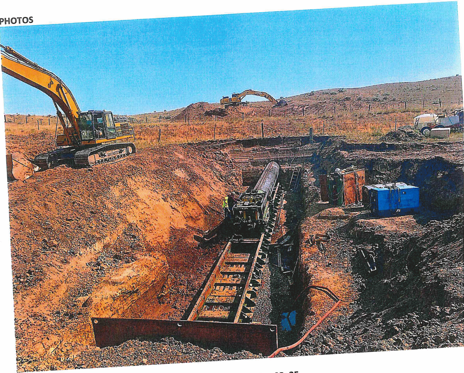
Coleman Construction Jack and Bore 48" steel casing at station 32+35
