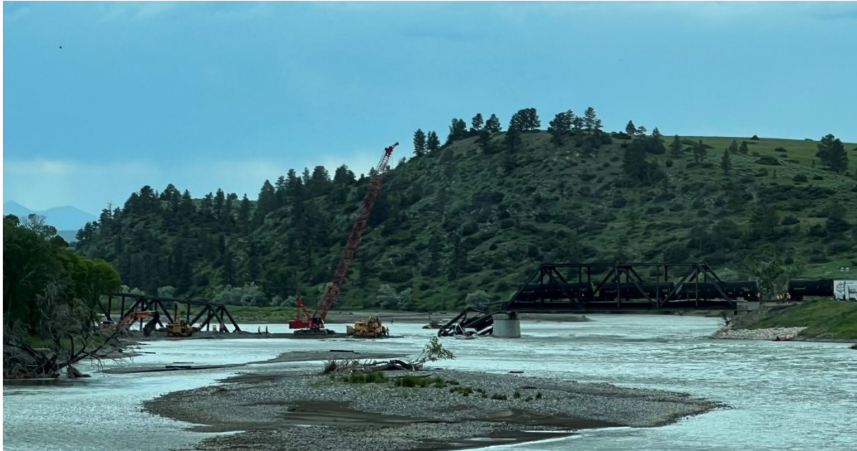
Figure 1-2. Side view of the Twin Bridges Road Railroad Bridge after the derailment.
