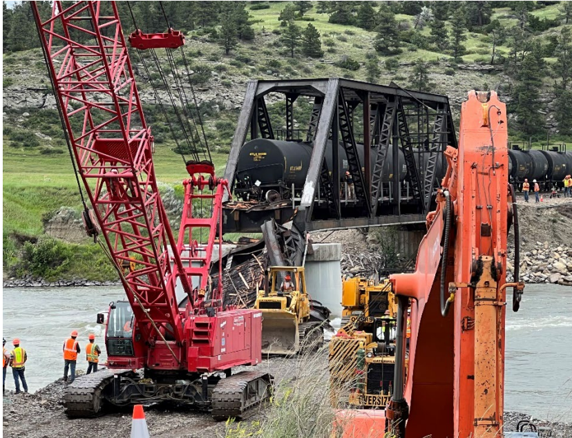
Figure 1-1. The Twin Bridges Road Railroad Bridge after the derailment.
