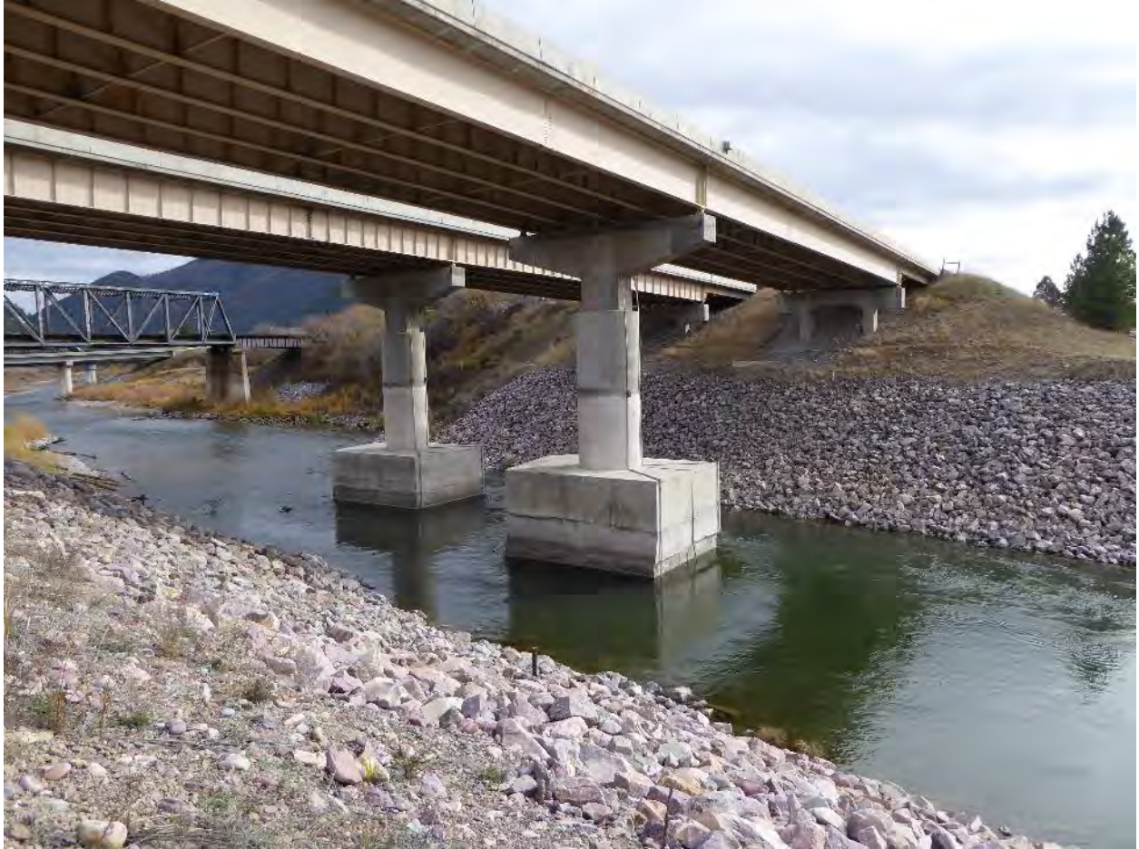
Riprap along the banks of the Blackfoot River under the Interstate-90 bridge.
