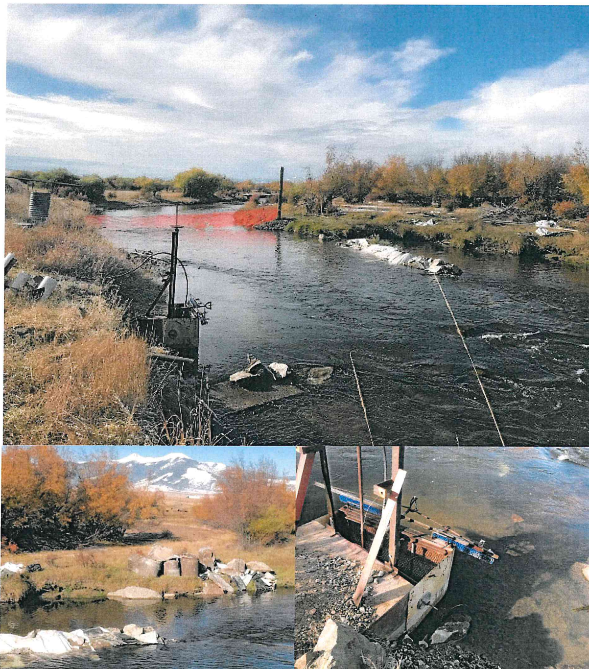
Figure 5 – Broken Circle Pumps Dam, push-up debris and intake with makeshift screen. Trout Unlimited Photos
