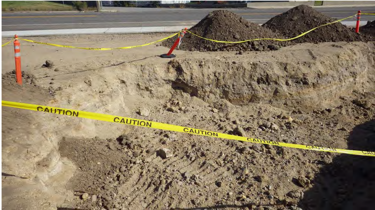
Photo 3. Tree pod excavation
