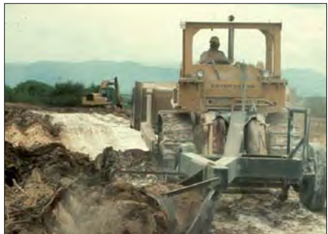
Deep plow tilling and incorporation of lime is an effective tailings remediation tool.
