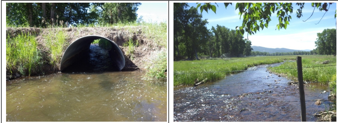
Undersized culvert with eroding road fill at Porters Corner Lane, F06
