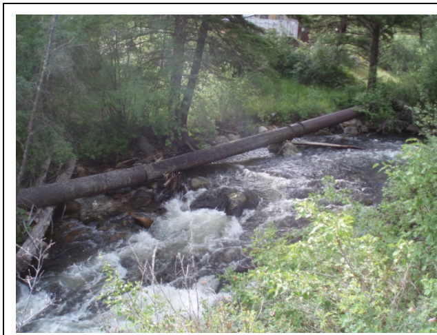
Old pipe suspended over stream runs along banks throughout reach in B09
