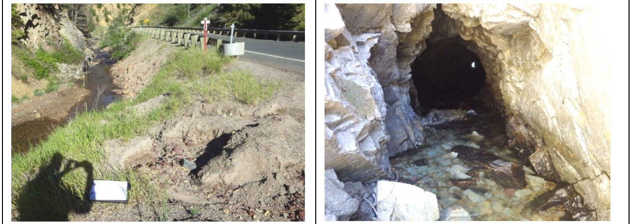
Confined channel and erosion of road fill from Hwy 1 in F01
