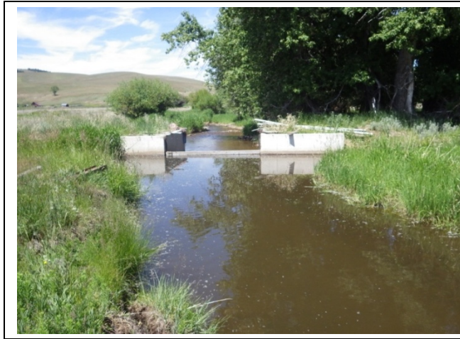
Diversion and eroding left bank at F07
