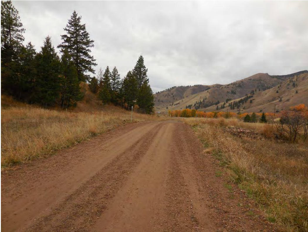
Photo #1 – View of roadway looking west over culvert.
