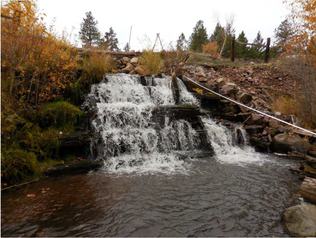
Photo #9 – View of existing timber fish barrier.
