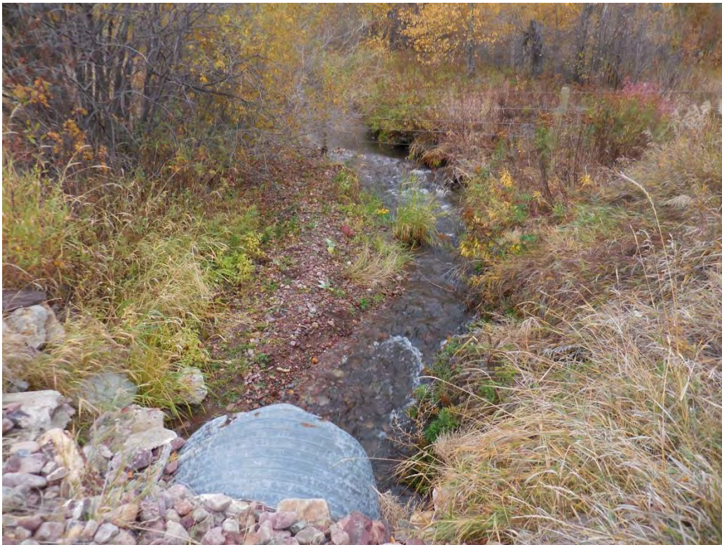
Photo #4 – View of Harvey Creek looking upstream from culvert inlet.
