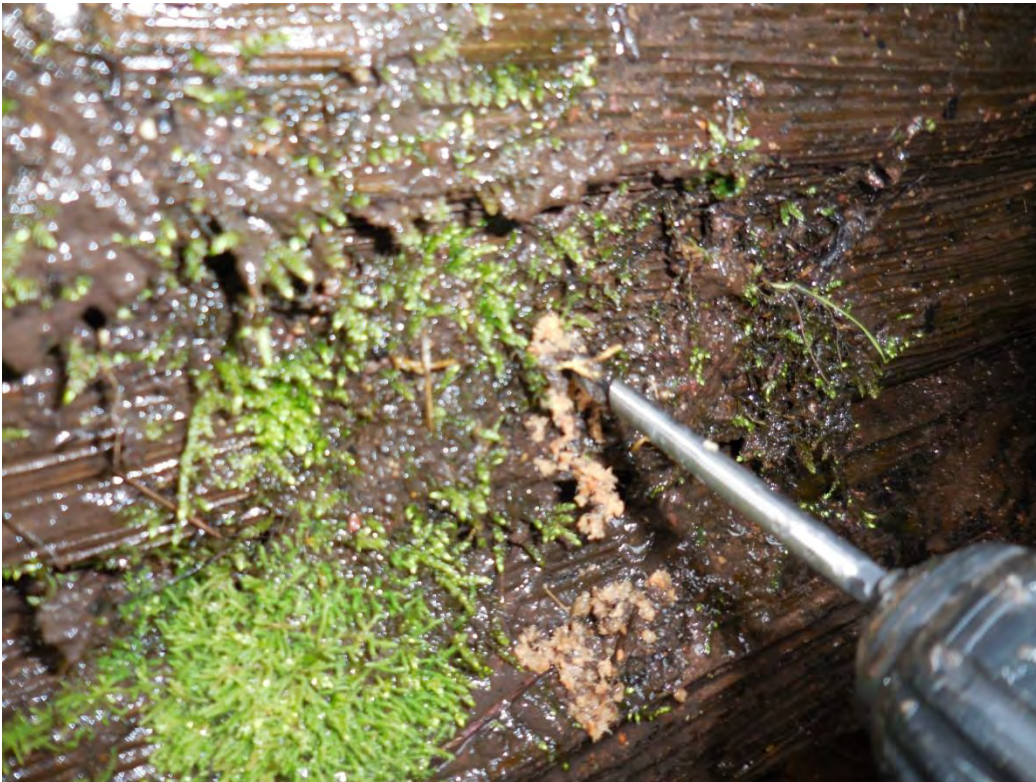
Photo #14 – View of timber coring taken on upper sill at west side.
