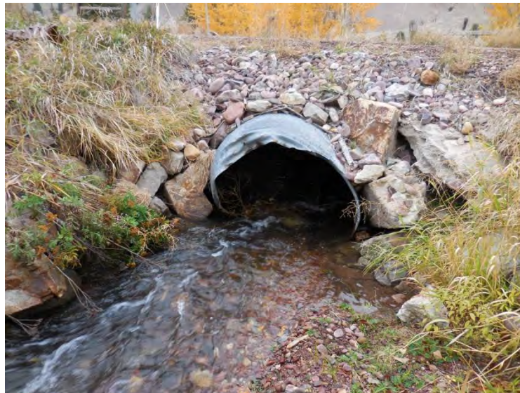
Figure 8: View of existing culvert inlet
