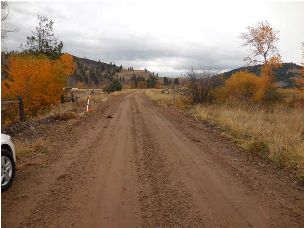
Photo #2 – View of roadway looking east over culvert.
