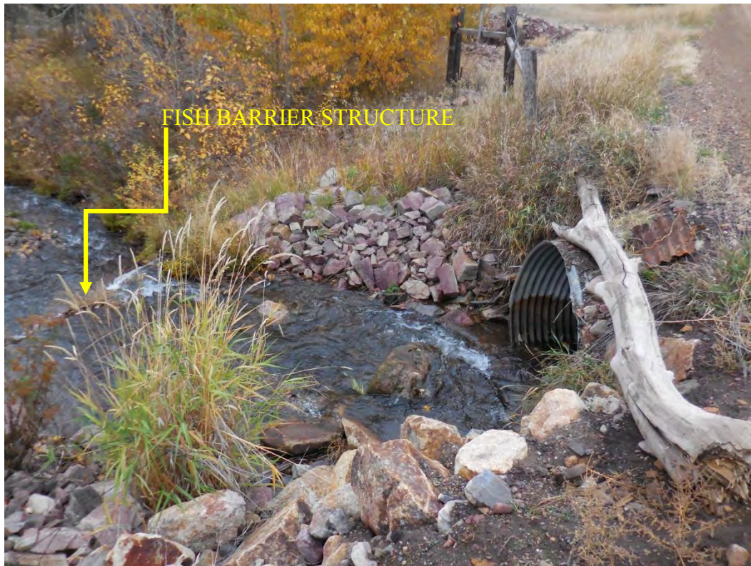
Photo #5 – View of culvert outlet and fish barrier.
