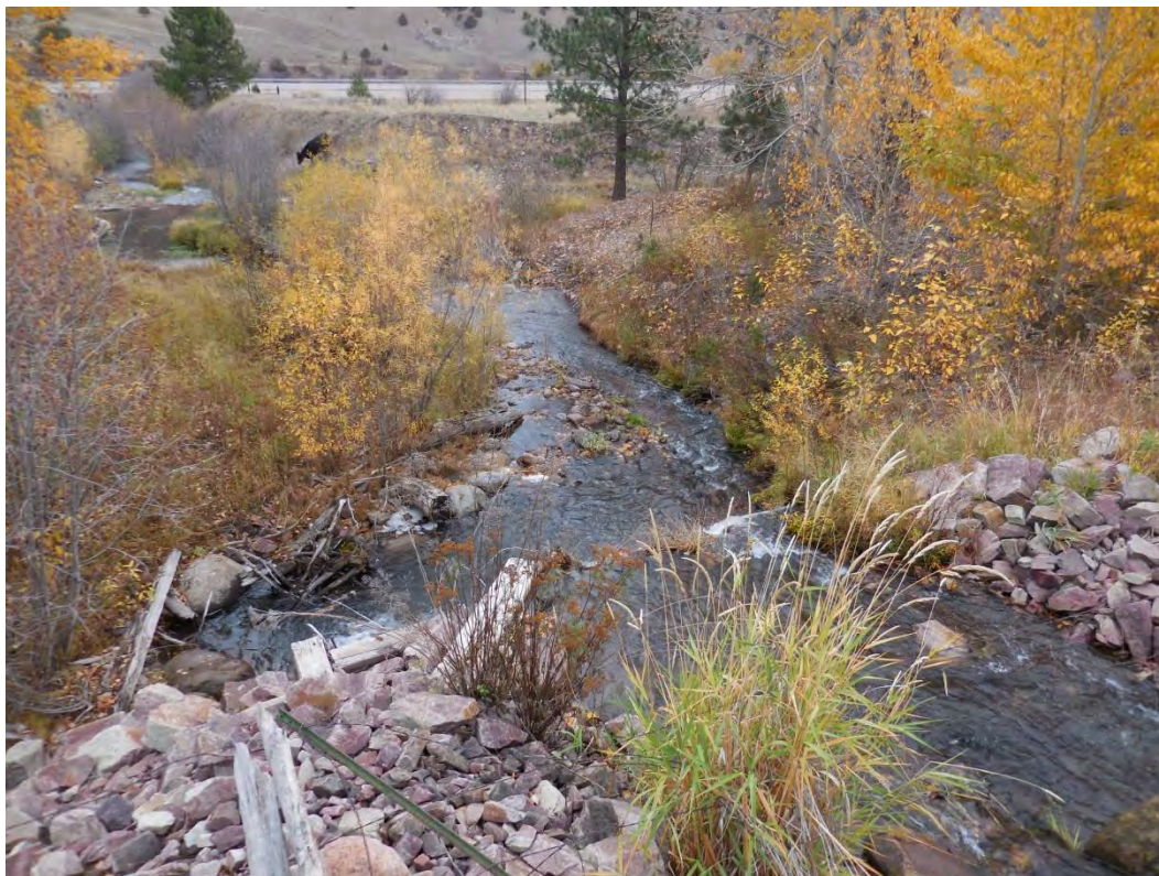
Photo #6 – View of fish barrier and channel looking downstream of culvert.
