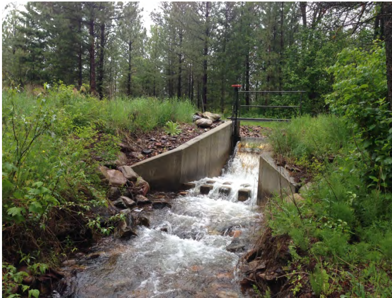
Figure 11: Cast-in-place concrete velocity barrier with dissipation
